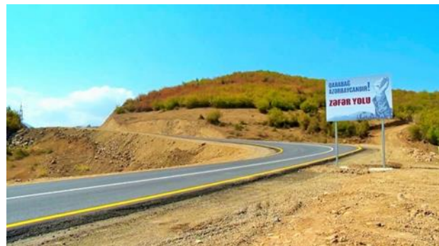
Figure 2. "Zafaryolu" after construction
